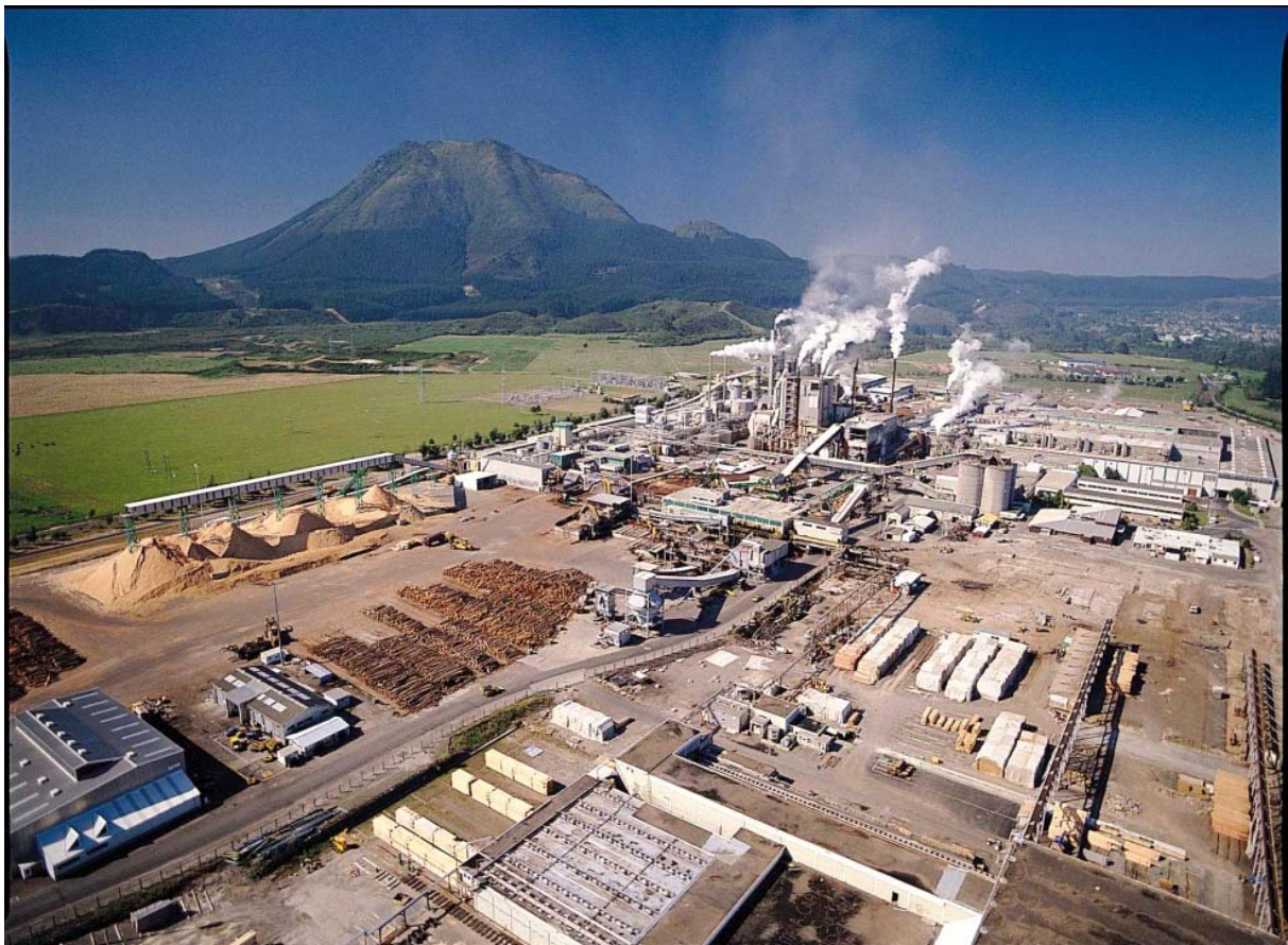
Photograph 3: Kawerau mill site, Bay of Plenty region. This is one of the largest geothermal direct heat uses in the world (5,316TJ/year), though use is now spread over three separate owners with supply from a fourth party.
