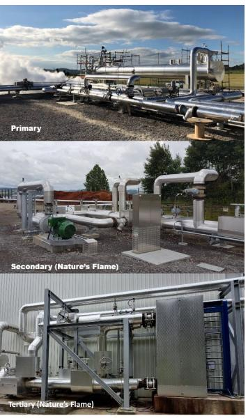
Heat is reduced through three heat exchanging loops (two heat exchangers) to supply 125°C clean hot water to the drier with 22MW of thermal energy available.
