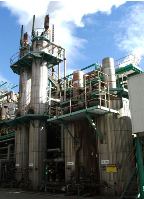
Photo of the plant at the Tasman Mill to de-gas the geothermal condensate producing feedwater. Two parallel process streams; two stripper vessels on the left and two flash tanks on the right
