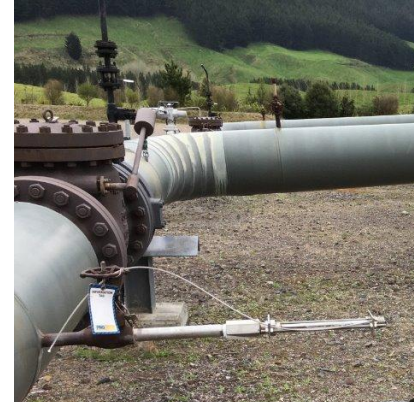
Corrosion Coupon *corrosion allowance ~3mm
