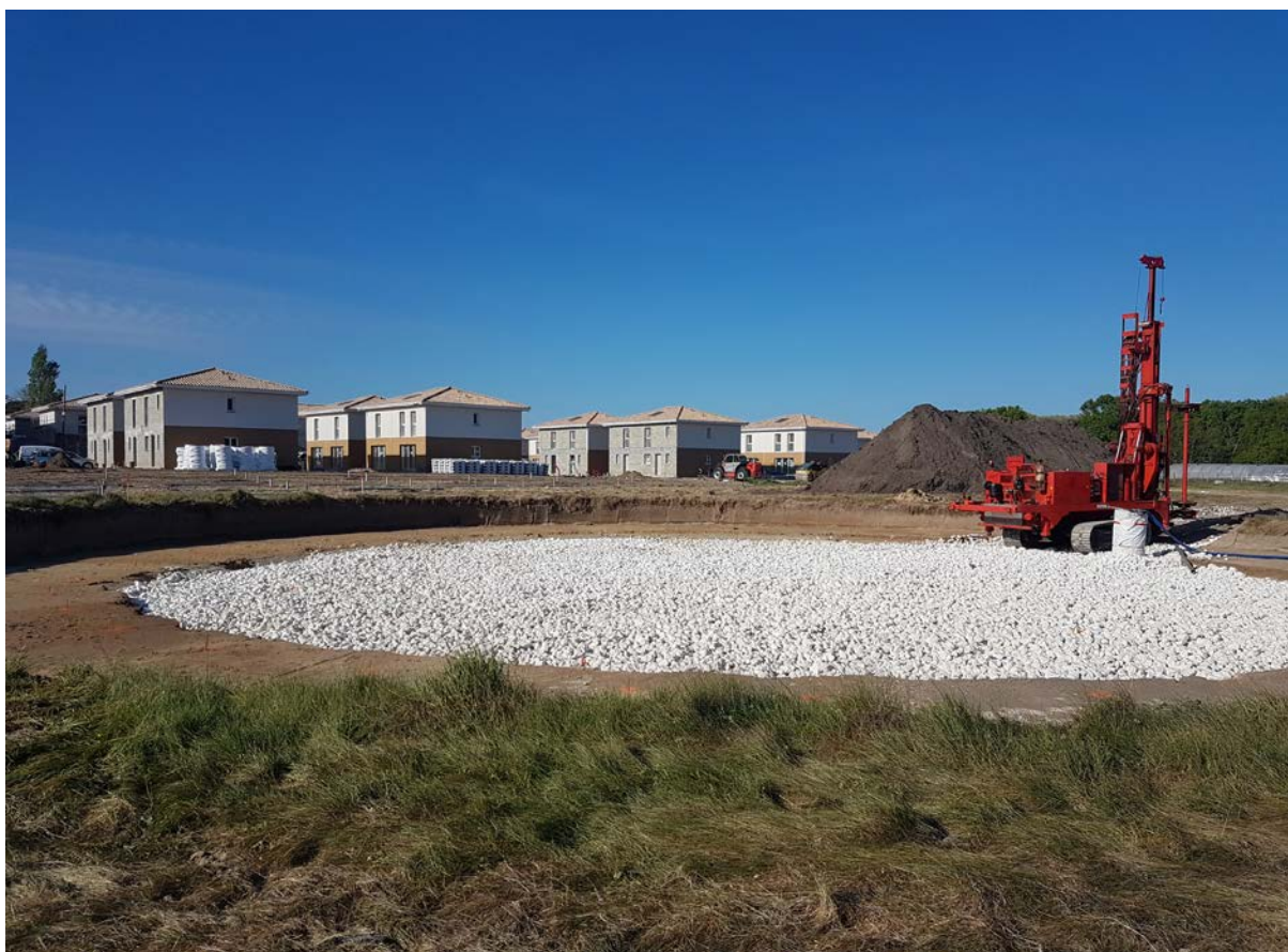
Figure 15 Top of the BTES awaiting cover placement
