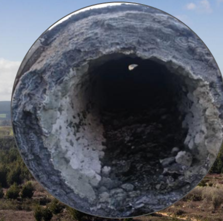
Pipe line upstream of Northern Plant
