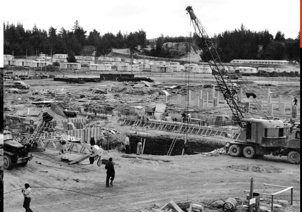
"Station 'A' Powerhouse 1/10/57. Electrical Annex left, outdoor station right, excavation to cable tunnel foreground"
