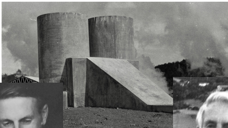
"Bore 42 23-11-56. Twin cyclone silencer".
