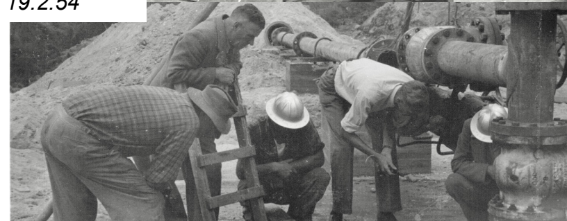
"Bore 26- Wellhead setup. 19.2.54"
