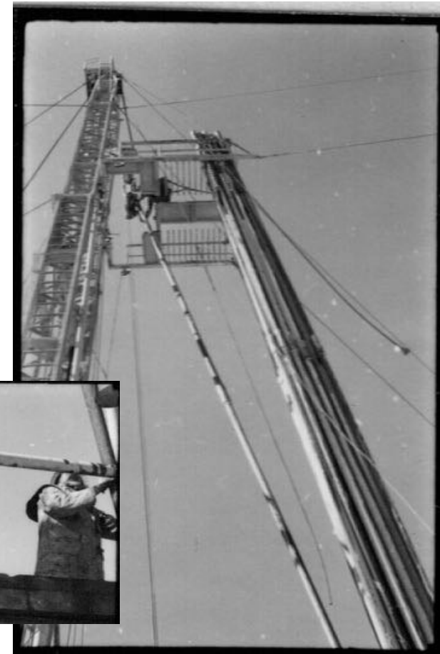
"Bore 25. 3.12.54. T12 rig running in drill pipe to get core"
