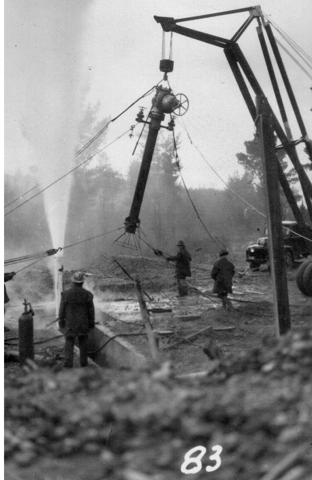
"Wairakei Geothermal Project. Bore No. 20. 16.5.53. Rigging up 10" valve & assembly"
