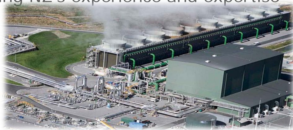
Nga Awa Purua (2010) – 140 MW, Triple Flash single steam turbine
