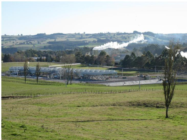
A binary plant uses geothermal steam and water to heat an intermediate liquid with a low boiling point to produce a vapour that spins gas turbines. This type of technology is particularly suited to plants using relatively low volumes of geothermal steam and fluid.
