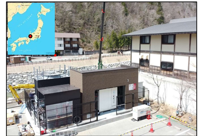
Baseload Power Japan, 50 kWe units at Midori, Japan. Midori #1: 307 l/min, 87 °C water, from ~45 - 50 m depth
